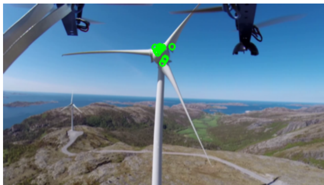
Fig. 5: The green circles show the points where the blade lines intersect each other.
